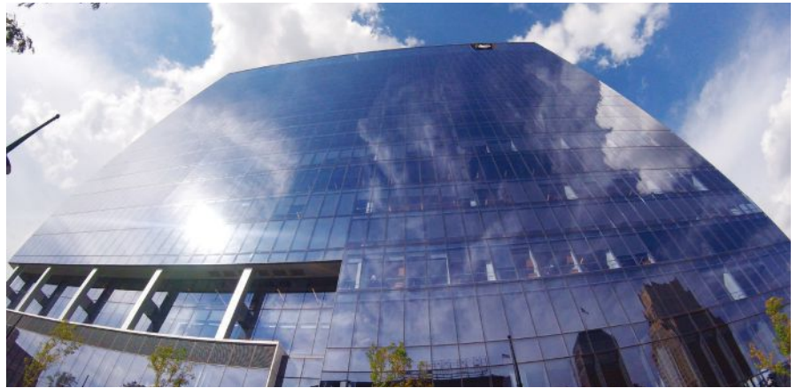
Window Film Depot’s latest installation, the Prudential Tower in Newark, N.J.
