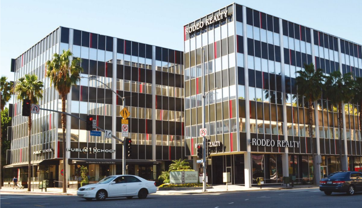
Solar Art installed exterior silver tint and red vinyl wrap accents on the Sherman Oaks building in Los Angeles, Calif.
